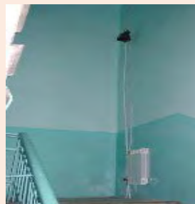
Installation of heaters
